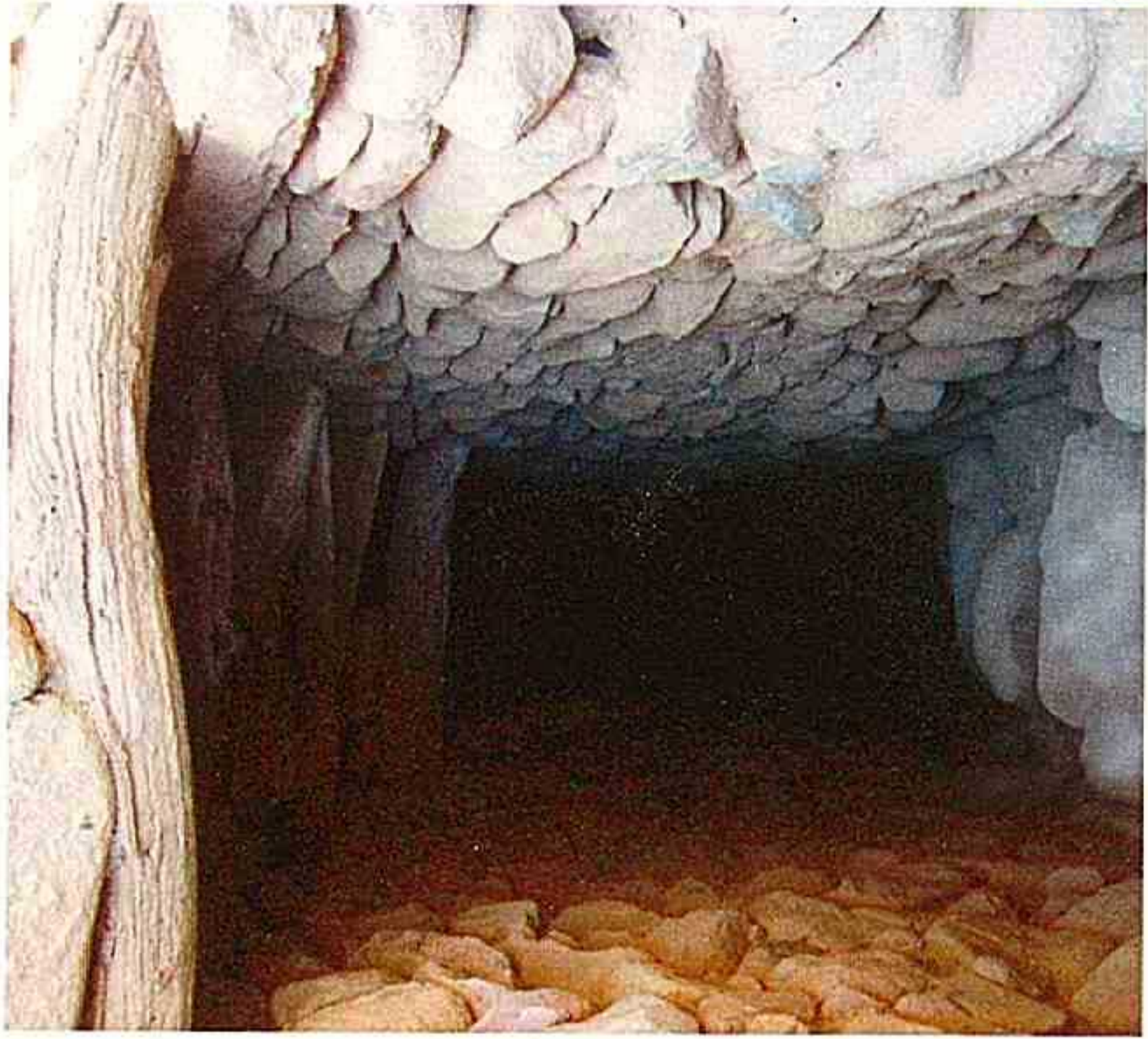
Picture 47. Entrance into forty-stepped built by river stone and baked brick in Ordubad city
